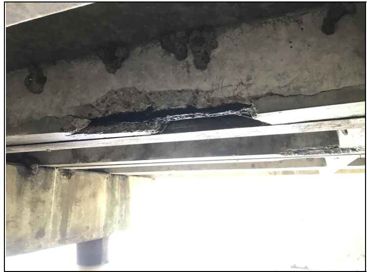
Spalls with rebar exposed to girders @ all spans. Some with section loss. (See Form III)
