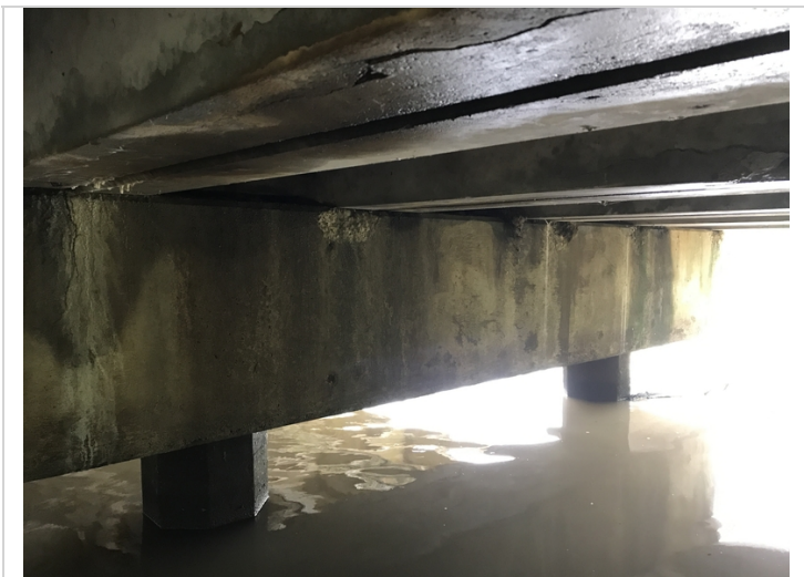
Spalls to ahead side of cap @ bent 17 @ girders 1 - 7.
