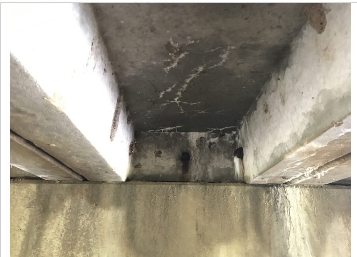
Efflor cracks to soffit @ girder 5.
