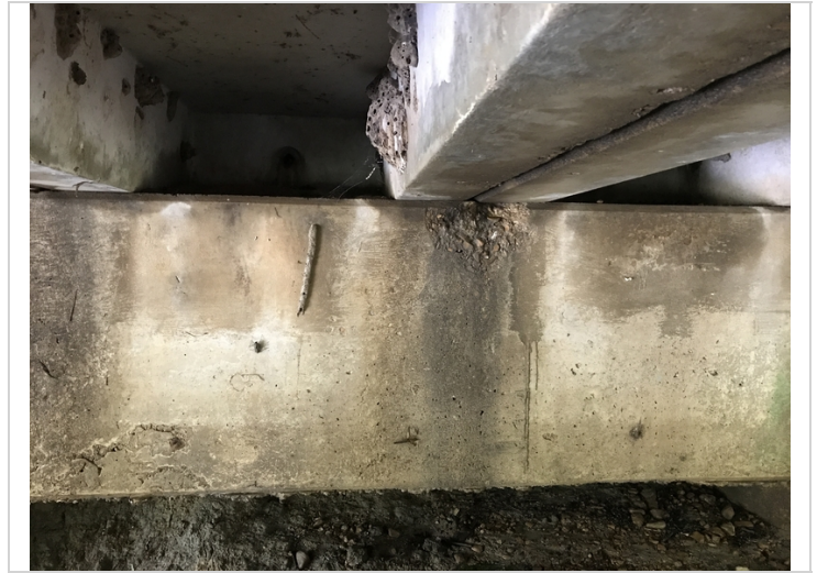
Spalls to abutment 2 with no rebar exposed @ girders 3 & 5.
