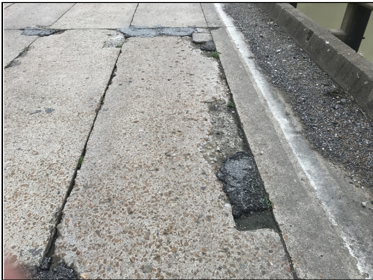
Spalls with rebar exposed to unit 6 @ span 1.
