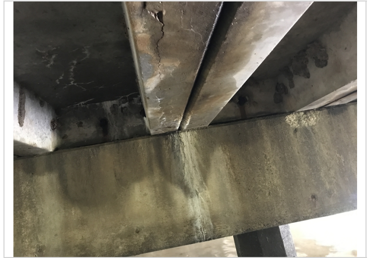
Areas of efflor cracks to girders @ all span.
