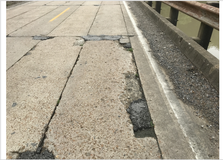
Typical spalls with rebar exposed to units @ all spans.
