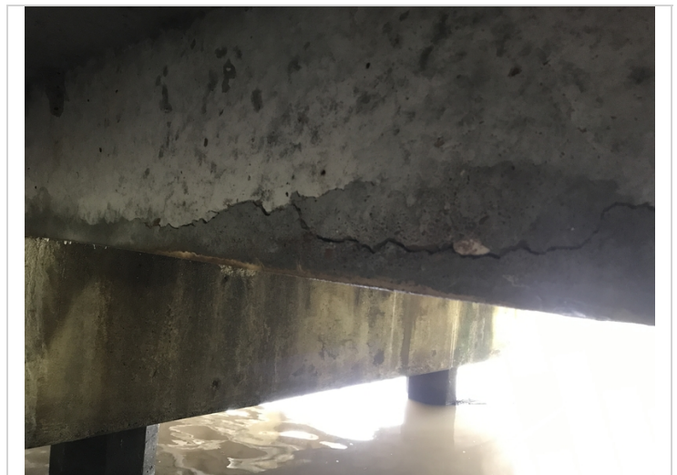
Typical cracks to girders @ all spans.
