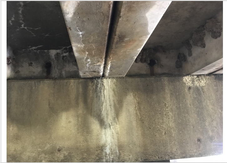
Areas of efflor to girders @ all spans.
