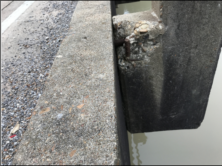
1st concrete guardrail post on Right side of Span 4, 5, 6 & 14 have spalls with rebar exposed. Span 5.
