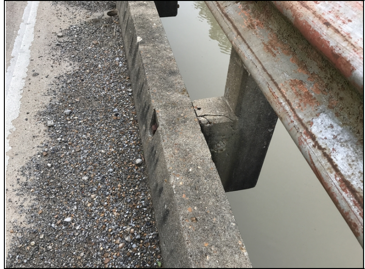
1st concrete guardrail post on Right side of Span 4, 5, 6 & 14 have spalls with rebar exposed. Span 4
