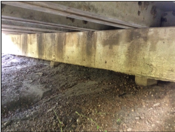
Undermining 1' down & 2' back under Abutment 2 with 3 piles exposed.
